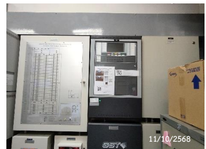
Fire Alarm Control Panel
