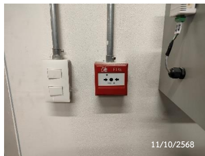
Fire Alarm Manual Call Point
